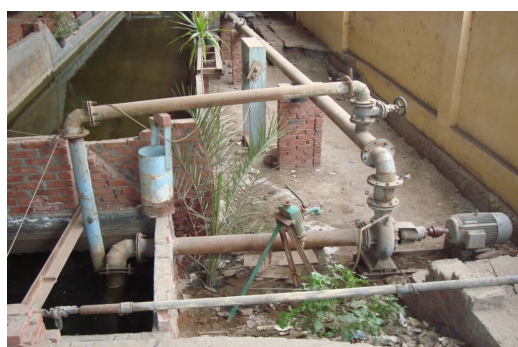
Photo 8. Feeding system of the side sump of the model (Front view)
